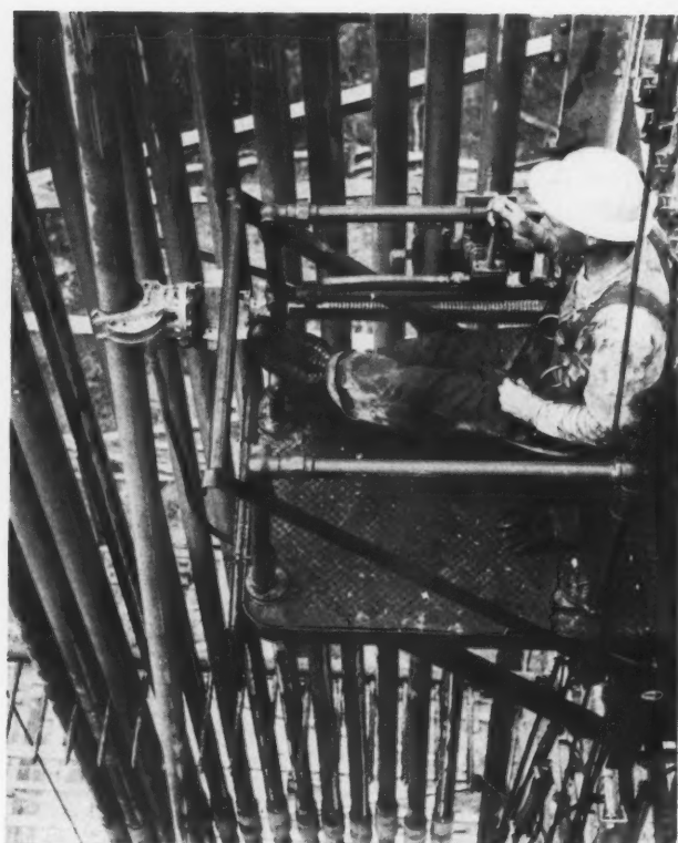
DERRICKMEN have long been accustomed to leaning far off the monkey board to steady the drill pipe as it is screwed up. NOW THE derrickman can rack many thousands of feet of drill pipe with no effort save tilting the control handle in his hand.
